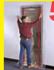
**5** Holding the ZipDoor sheet at the top, place it so the sheet is centered on the doorway. **Important: Leave two to three inches of sheeting to overlap at the floor.** This limits dust from coming under the door. Press sheet against tape.
