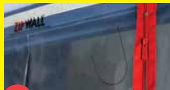
**6** Install the enclosed Flap Hooks for holding up the door flap when easy access is needed. On the back of the flap, poke the short end of the hooks through the plastic sheeting just below the top of the doorway and let them hang there ready for use.
