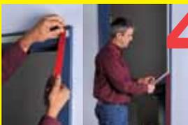
**4** Apply ZipWall® Tape to the left and right sides of the doorway. **Be sure to overlap with tape at the top to create a continuous seal around the door.** Then remove the red release-paper.
