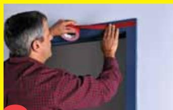
**2** Apply ZipWall® Tape at the top of the doorway. The low-tack adhesive faces paint, high-tack adhesive is covered by red release-paper.
