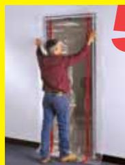
**5** Holding the ZipDoor sheet at the top, place it so the sheet is centered on the doorway. **Important: Leave two to three inches of sheeting to overlap at the floor.** This limits dust from coming under the door. Press sheet against tape.
