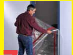
**7 To remove:** Carefully peel the tape and plastic off the doorframe. To minimize paint damage pull the tape off slowly.
