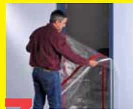
**7 To remove:** Carefully peel the tape and plastic off the doorframe. To minimize paint damage pull the tape off slowly.
