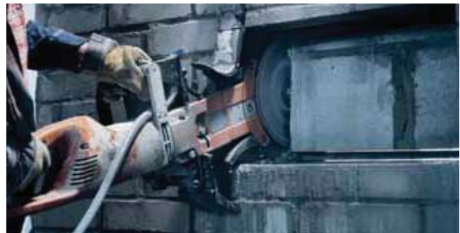
Efficient electric cutter with convenient method for cutting up to 16" deep.
