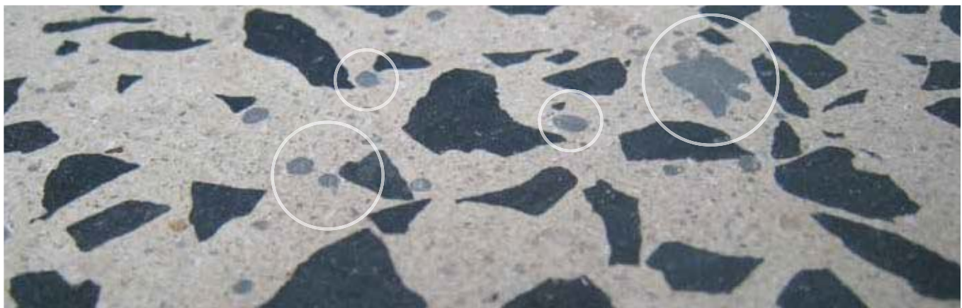
Holes filled when grinding with 120 grit metal-bonded diamonds and GM 3000™.
