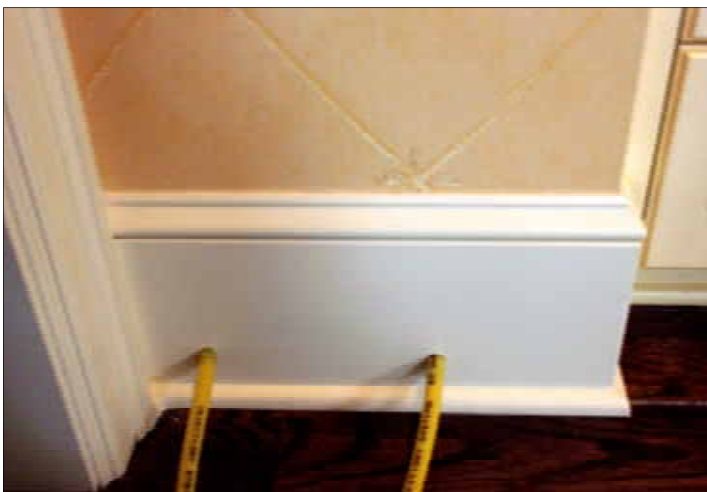
INJ01 drying walls through 1/4" easy to repair holes in baseboard in order to save wallpaper
