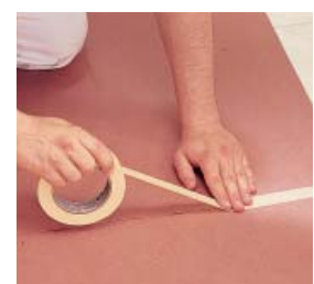
Taping paper to protect floors
