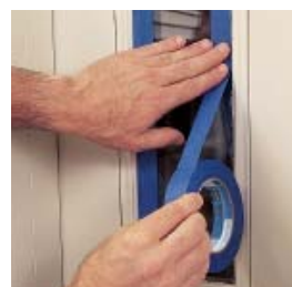
Masking exterior glass
