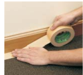
Masking baseboard to protect floor
