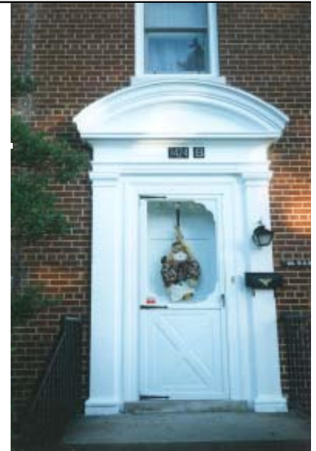
Figure 4. L-B-C over wood door frames at Fort Knox, KY
