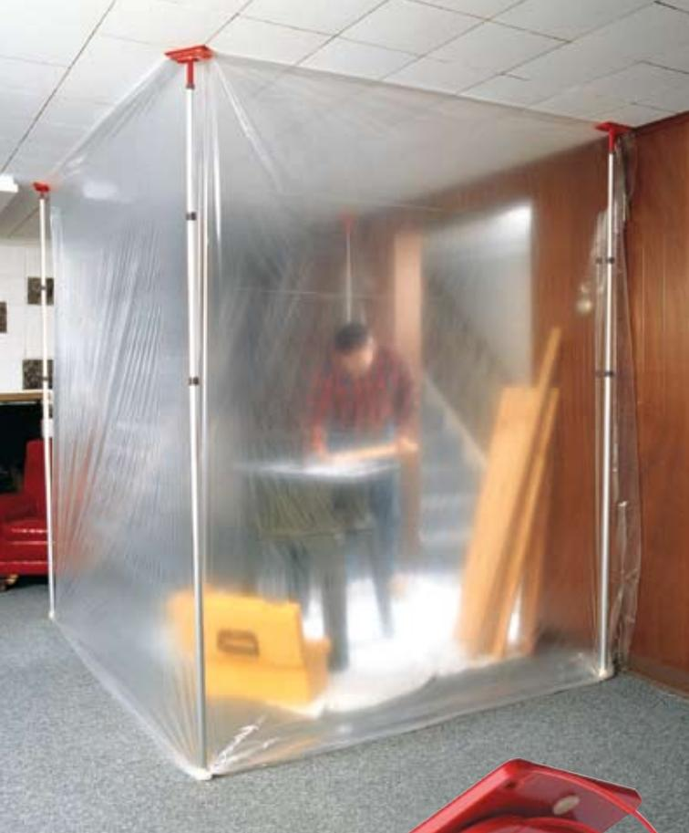
***This three sided plastic dust barrier was put up by one person in less than five minutes.***
