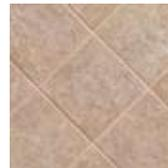
A key advantage of ceramic flooring is its durability. Ceramic is resistant to alkaline, acids and solvent used in cleaning. Ceramic's abrasion resistance keeps it from being scratched by gritty soil under foot if the grade of tile matches the situation in which it is used. Ceramic flooring is available in a wide variety of styles, colors and patterns
